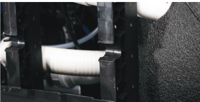
French Cleat (top) and C-Clip (bottom)
